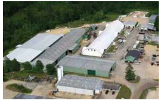
Laminating Plant - El Dorado, AR
